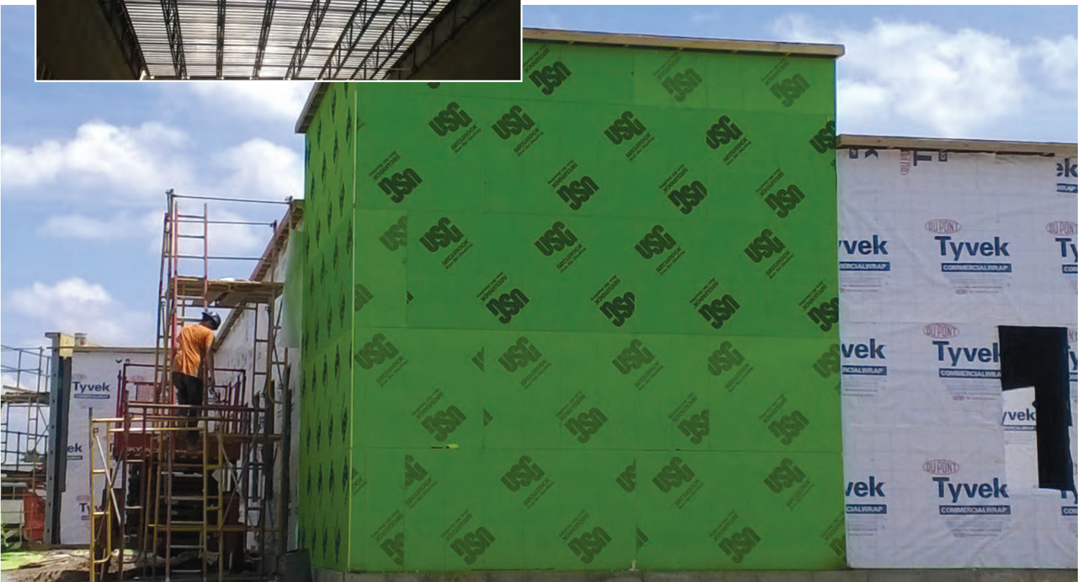
Below: The corner panels for the new wing are up.
