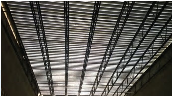
Left: The ceiling is in place for the new Gymnasium.
