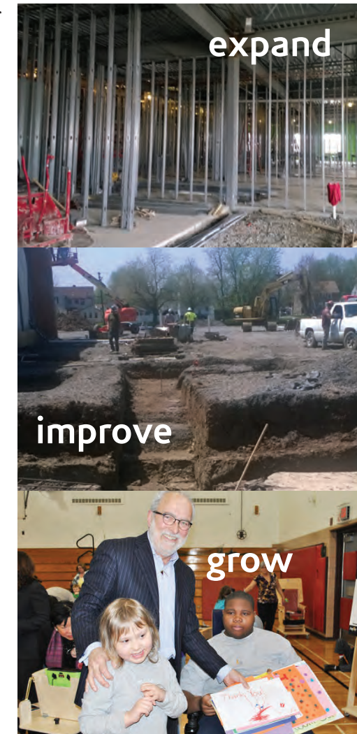
Top: Space being created for the new administrative wing.
